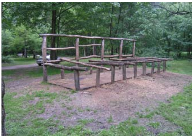
Figure 9.22. A semi-primitive tie stall design that is working in part because the stall floors are standard stall mats. This particular structure is made of black locust, the only wood in eastern North America sufficiently hard to withstand chewing by horses. It is also naturally rot and termite resistant. (Photo by G. W. Wood.)
