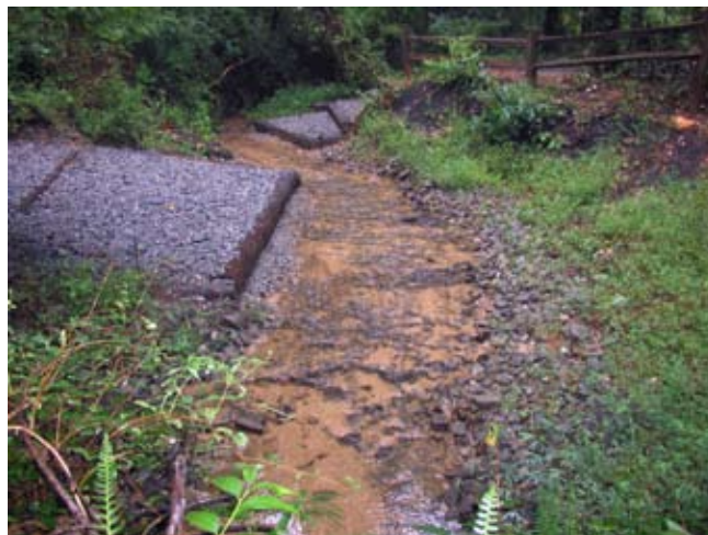
Figure 9.7. A hardened watering site that will withstand substantial heavy use without suffering streambank or streambed degradation. (Photo by G. W. Wood.)
