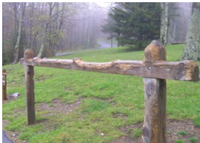
Figure 9.23. A heavily chewed, pressure-treated, 4x6 pressure-treated southern pine hitching rail that has lost much of its functional integrity in terms of strength. (Photo by G. W. Wood.)
