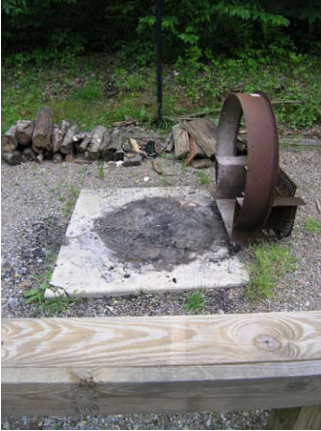
Figure 9.14. Fire ring hinged into post set into concrete slab. (Manufacturer: Pilot Rock Park Equipment, R. J. Thomas Mfg. Co., Cherokee, Iowa.) (Photo by G. W. Wood.)
