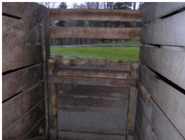
Figure 9.33. This covered stall is so narrow that access to a horse that was down would be both difficult and dangerous. (Photo by G. W. Wood.)
