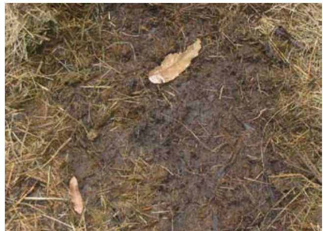
Figure 9.27. An accumulation of muck on top of the geoweb-quarry screening fill surface. Drainage rate might be increased by increasing the size of the fill material to a 4-6mm gravel. (Photo by Jeff Sprites.)
