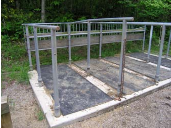
Figure 9.19. Horse tie station at Harmons Den, Pisgah National Forest, North Carolina (left) and a modification of the design at Great Smoky Mountains National Park, Tennessee (right). (Photo by G. W. Wood.)
