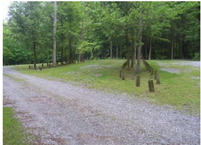
Figure 9.2. A pull-through parking design with spaces 45 ft. wide and 85 ft. long. This design offers substantial convenience to users that may tie horses to trailers for tacking, but it is very inefficient in the use of space as about 40% of the area is devoted to driveways. (Photo by G. W. Wood.)
