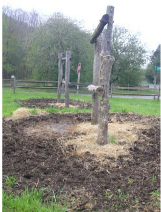
Figure 9.25. A hitching rail designed and heavily used for overnight tying. This is an alluvial soil that receives 45-50 in. of precipitation annually. The timbers have held up against rot and chewing because they are black locust; however, the ground surface is a mudhole in rainy periods. (Photo by G. W. Wood.)
