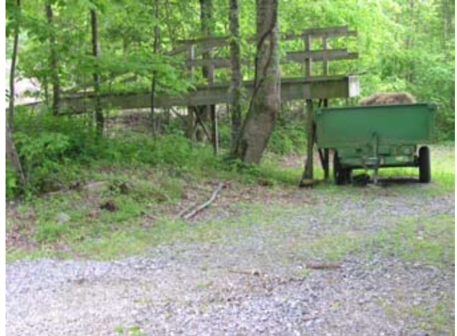
Figure 9.15. Manure management facility at Harmons Den Campground, Pisgah National Forest, North Carolina. (Photo by G. W. Wood.)
