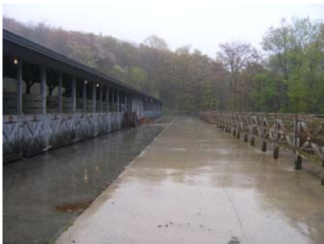
Figure 9.32. Covered stalls on left and open stalls on right at Grayson Highlands State Park, Virginia. These hardened surfaces will not provide a good opportunity for the horse to rest its legs. (Photo by G. W. Wood.)
