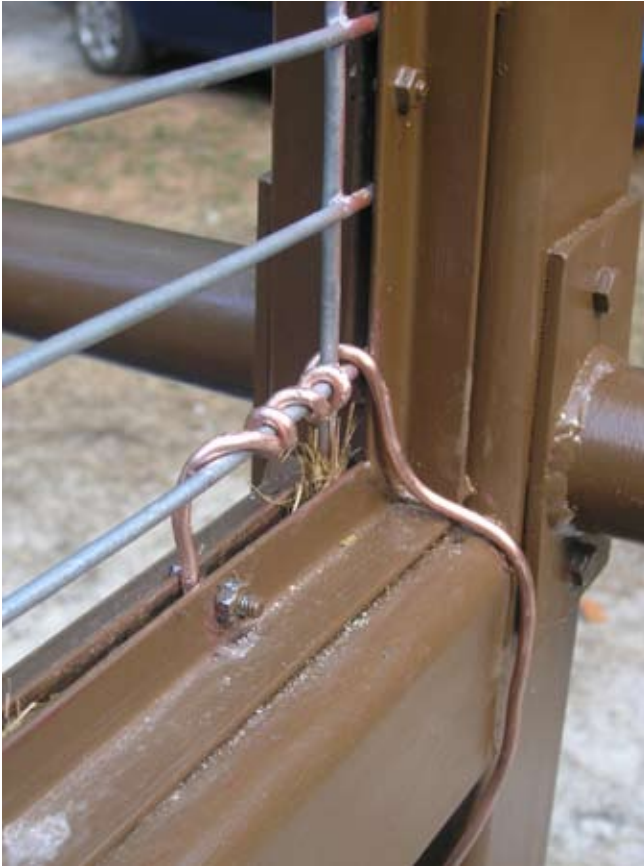
Figure D.10. Ground wire wrapped to central divider screen (left) and grounded to \frac{3}{8} -in. diameter copper ground rod driven 8 ft. into the ground (right). (Photo by G. W. Wood.)
