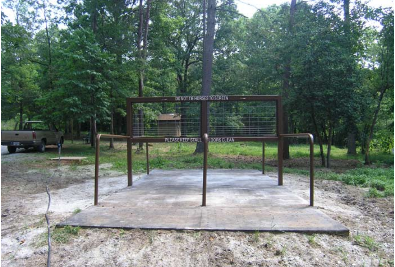
Figure D.2. The Clemson 4-Horse Tie Stall design. (Photo by G. W. Wood.)
