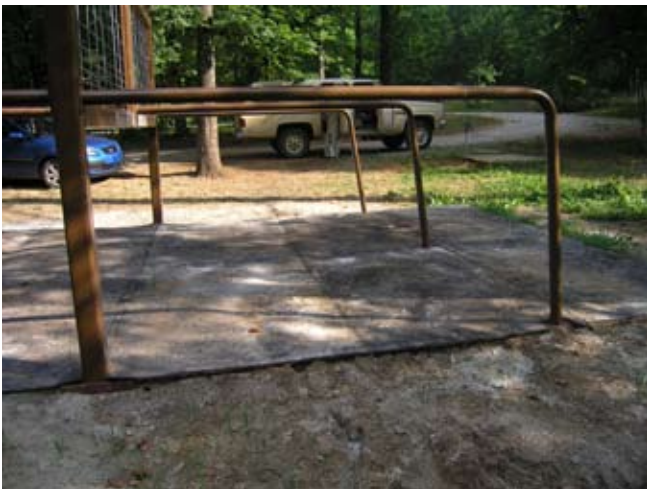
Figure D.8. Stall bars shaped by bending a 2-in diameter, schedule 40, iron pipe. The bars are 42 in. at the top line and extend 72 in. along the stall floor. (photo by G. W. Wood.)
